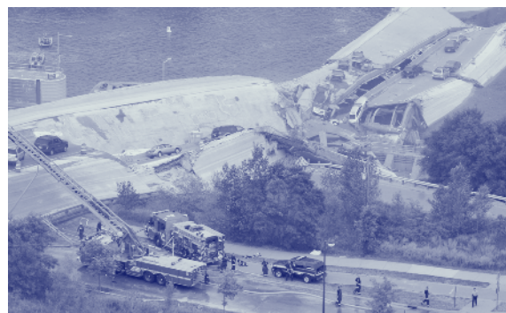
I35W bridge collapse
